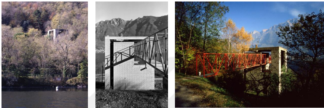
Figure 2.11. One of the houses that Mario Botta designed in Riva San Vitale, Switzerland, in 1971, with respect to the landscape conditions of the context and referring to a local summer-house type (Source: web 6).
