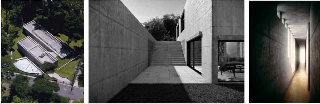
Figure 2.13. Koshino House in Japan by Tadao Ando who prioritizes local light and architectural details, which reinforce the tactile experience in his buildings (Sources: web 8 and 9).
