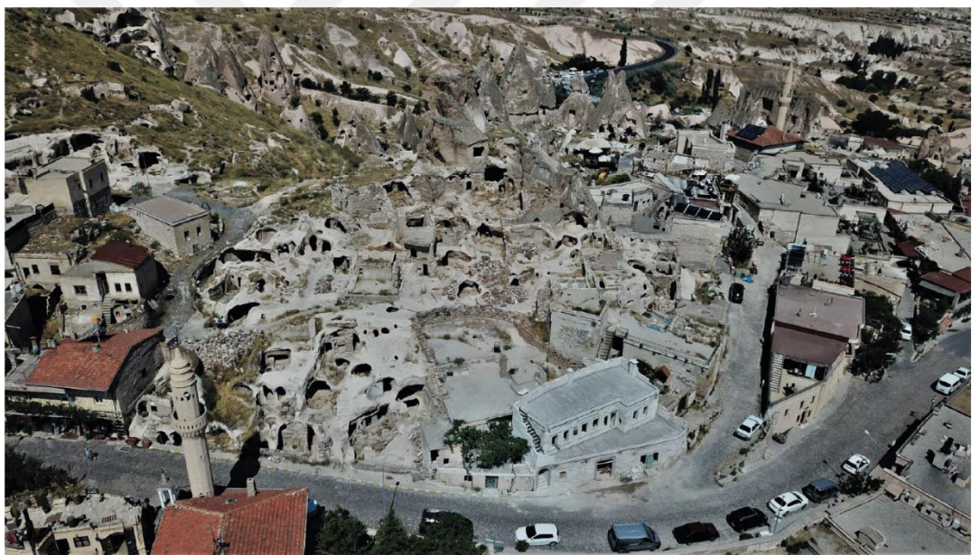
Figure B.14 Aerial photos of the plots (By courtesy of Argos Yapı, 2019)
