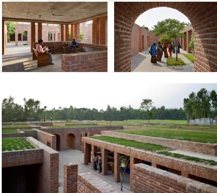
Figure 2.15. The Aga Khan Award recipient Friendship Centre project in Gaibandha/Bangladesh by Kashef Chowdhury. This building complex was completed with a rather limited budget. The designers had to react to the potential geographic problems such as flood in a subtle and economical manner. In terms of its tactile and tectonic character, the building refers to the close-by remains of an ancient town and employs only the local and hand-made bricks (Source: web 11; Alarcón, 2013).
