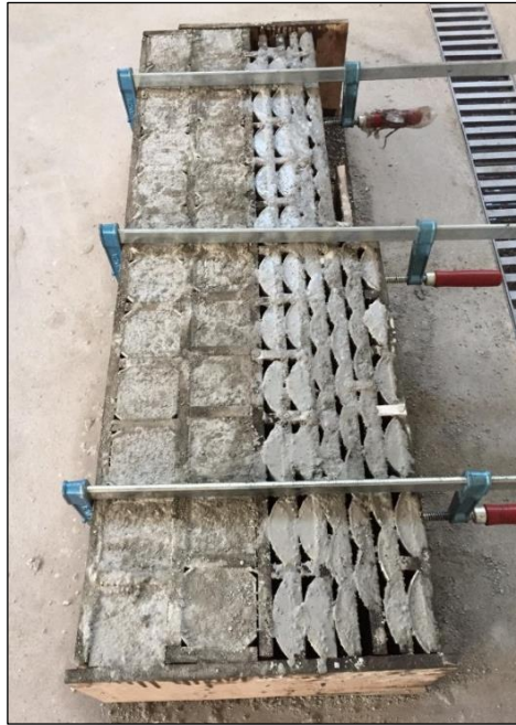
Picture 3.2. The formwork after casting the concrete
