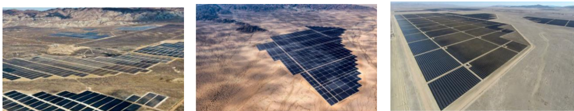
Figure 2. 9. Examples of SPP in California (Source: Webpages)
