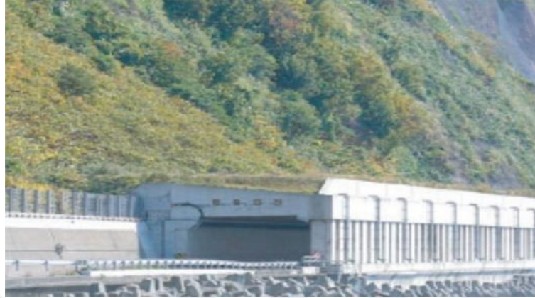
Figure 4.6. Sand pad use in rock protection tunnel [111].
