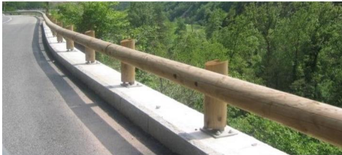
Figure 2.3. Wooden element guardrail [1].
