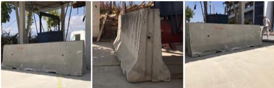
Figure 5.16. Concrete barrier installation to the crash point of pendulum system.
