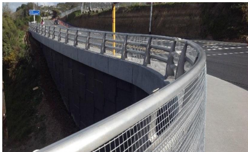
Figure 3.5. Steel tubular bridge barrier [75].
