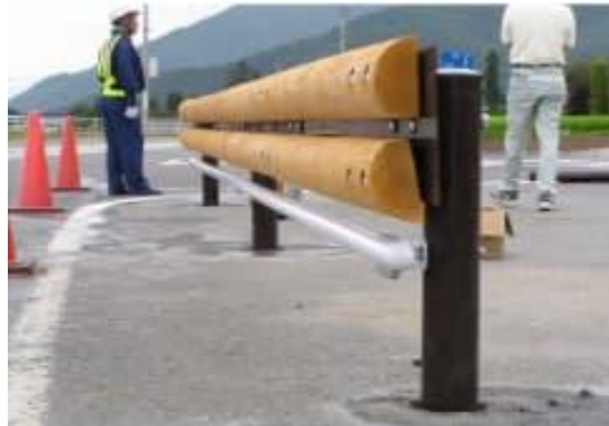
Figure 2.1. Steel post timber barrier [56].
