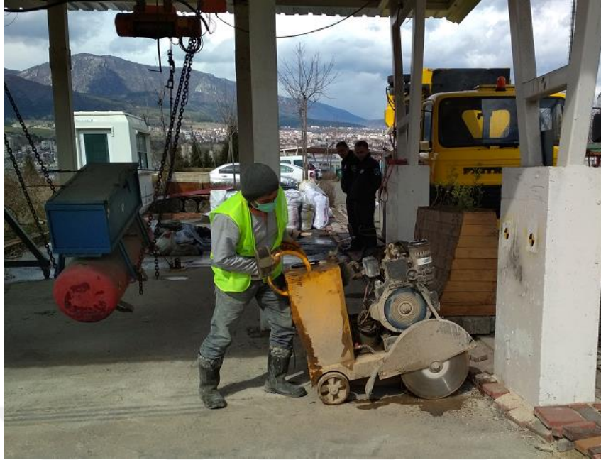
Figure 5.17. Concrete cutting machine.
