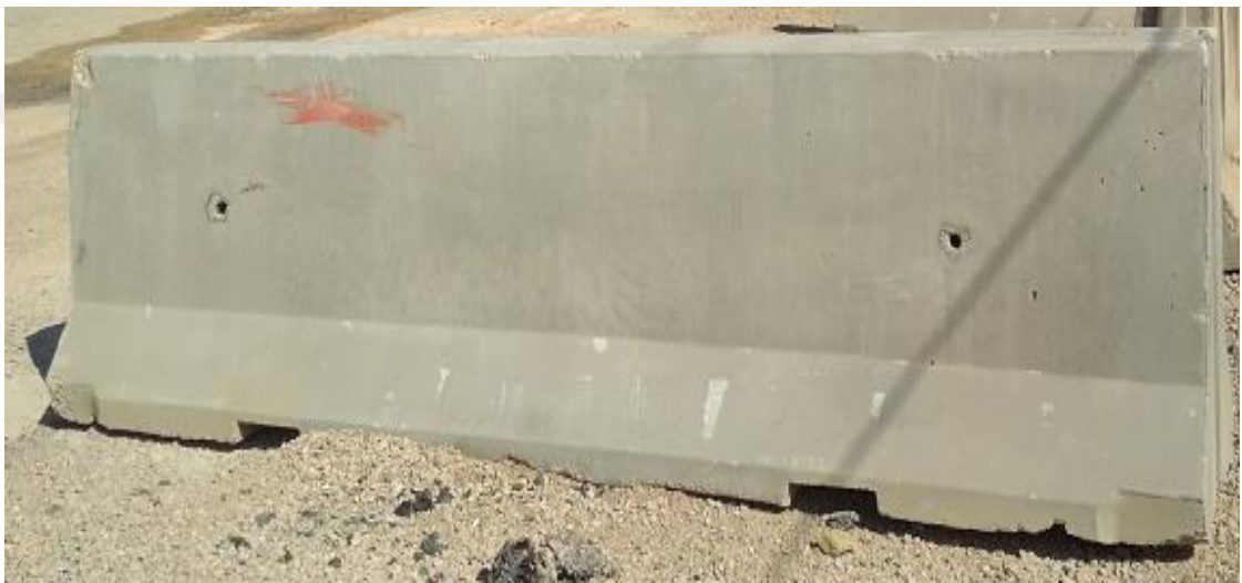
Figure 4.9. Concrete barrier shape
