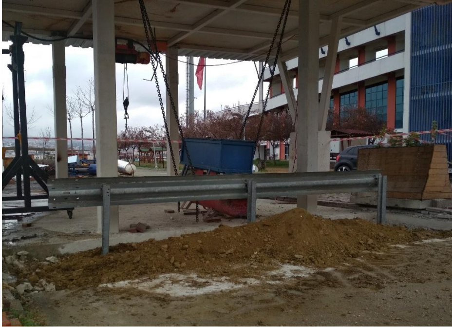
Figure 5.19. W- beam steel barrier after installation process.
