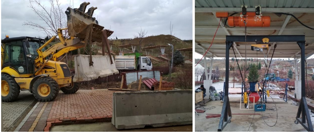
Figure 5.15. The installation process of the concrete barriers
