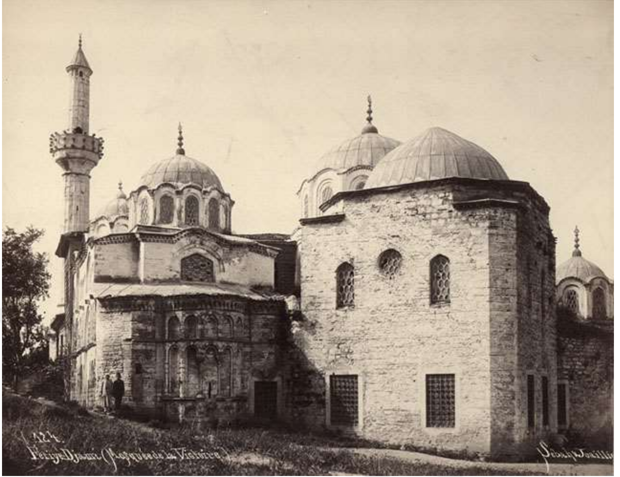
Figure 27: View of Fethiye from southeast with its minaret, photo by Sébah-Joallier Studio. 208
