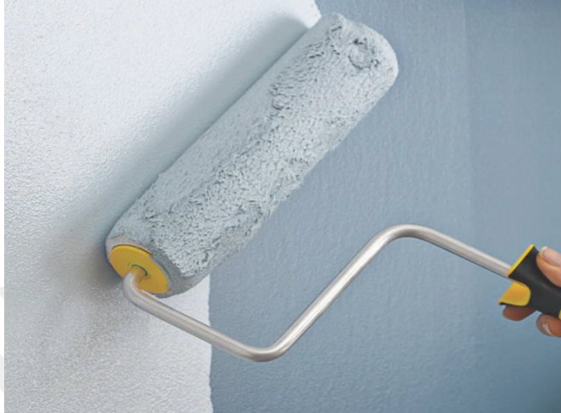
Figure 2.8. Roller Application of Painting
