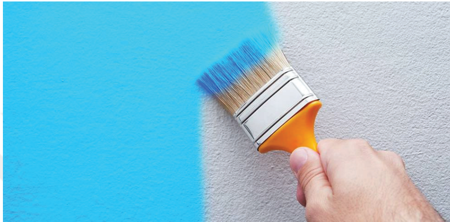
Figure 2.7. Brushing Application of Paint
