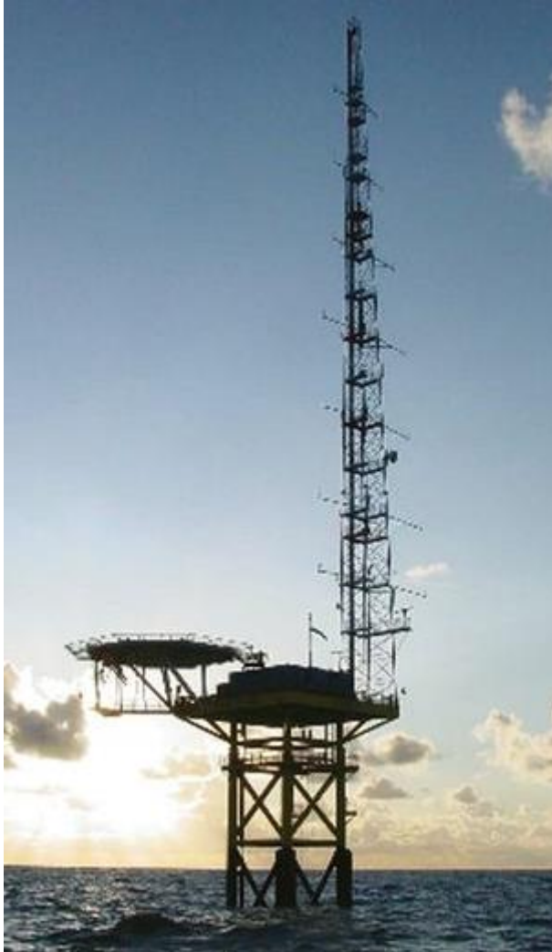
Figure 1.7. FINO-I platform with measurement mast that is ~100 m
