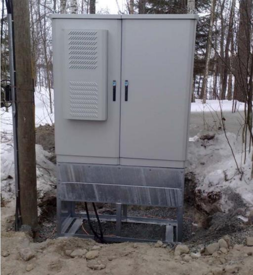
Figure 4.2 : Converter Cabinet Installation at the Site [21]
