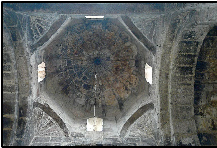
Figure 3.32. Odzun Basilica's dome, supported by 4 squinches, Armenia [82]
