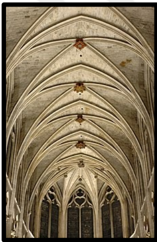
Figure 1.9. Masonry vault, Saint-Séverin Church, Paris, France [16]
