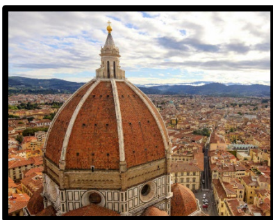
Figure 1.10. Masonry dome, Santa Maria del Fiore, Florence, Italy [17]
