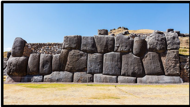
Figure 3.1. Rubble masonry, Sacsayhuaman, Cusco, Peru [54]
