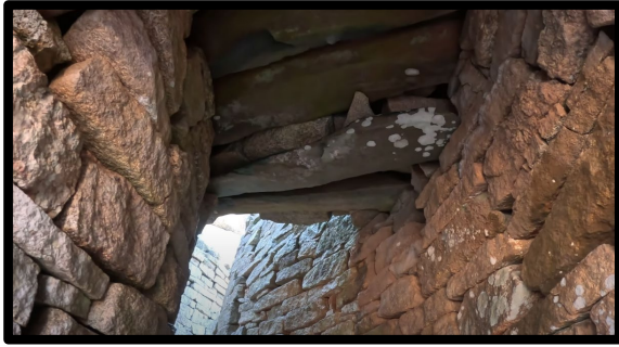
Figure 3.10. Example usage of flat stones as beams [57]
