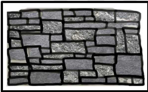
Figure 3.4. Ashlar masonry wall exterior view
