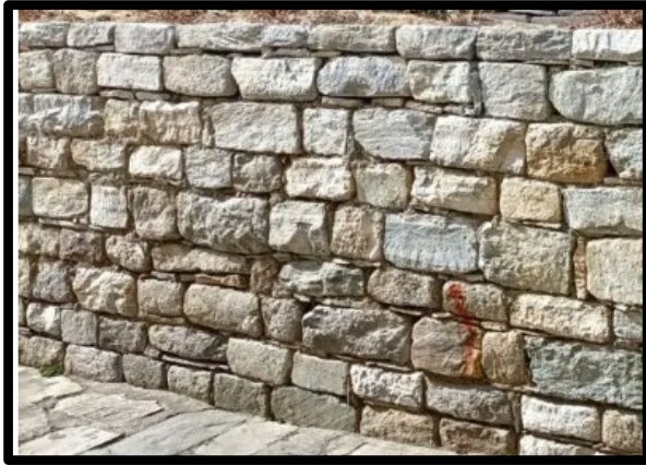
Figure 3.5. Coursed rubble masonry [56]
