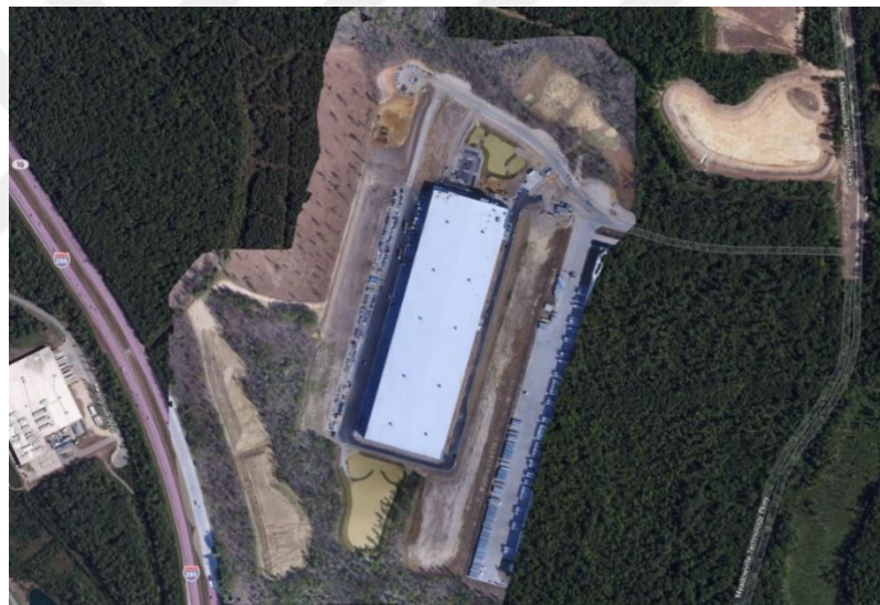
Figure 3.15. Manufacturing plant construction site: drone mapping (Drones for Construction Project Management eBook, 2017).
