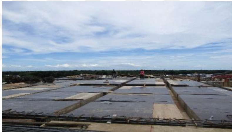
Figure 3.6. Construction site image captured by a common digital camera (Kaamin et al, 2017).
