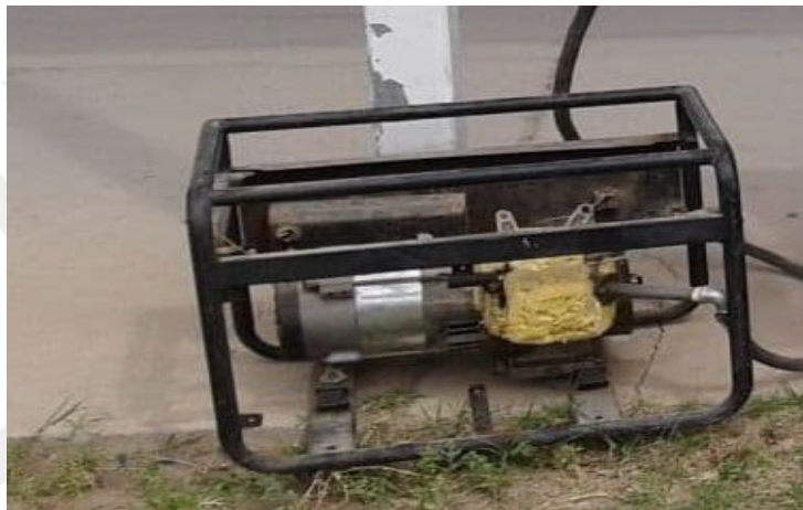
Figure 3.14: Electric generator view after modification.
