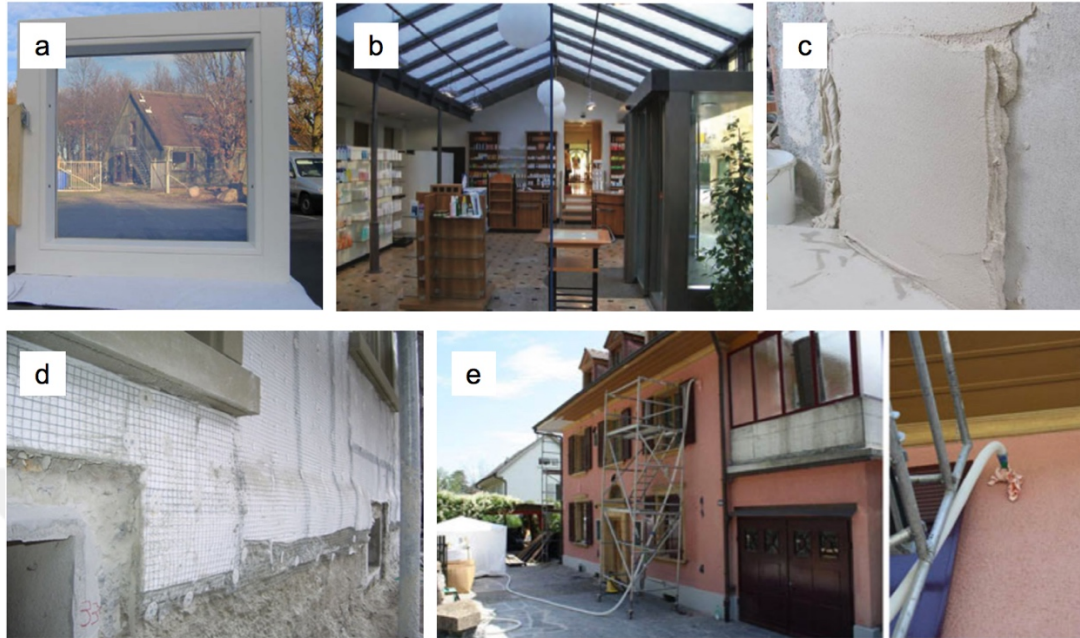
Figure 6 Photographs of (a) aerogel glazing, (b) the translucent aerogel roof, (c) render system, (d) the wall and window sill detail from the retrofit insulation with aerogel blankets, (e) the injection hole for cavity wall insulation (Koebel et al., 2012; Riffat & Qiu, 2013)
