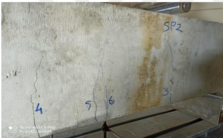
Figure 4.33 Crack formation of the initial stage of the experiment
