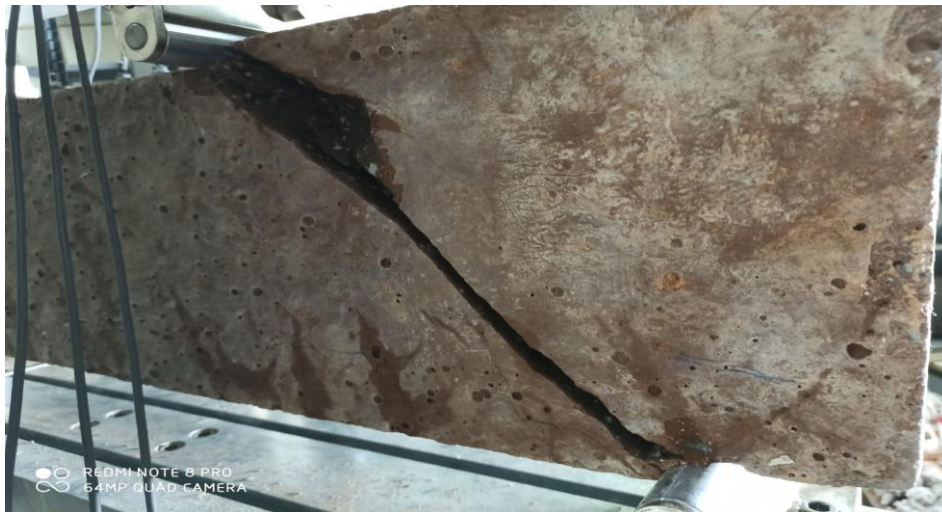
Figure 4.13 10 mm wide shear crack formation in the posterior between supports
