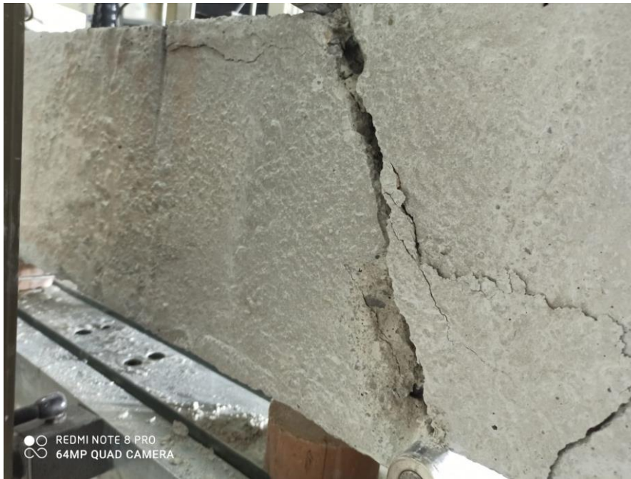
Figure 4.29 Large shear crack at the back of the specimen after the test
