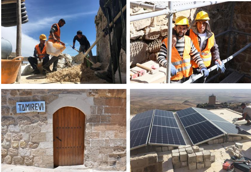
Figures 5.48- 5.51: Tamirevi and its construction process (KMKD, 2020).
