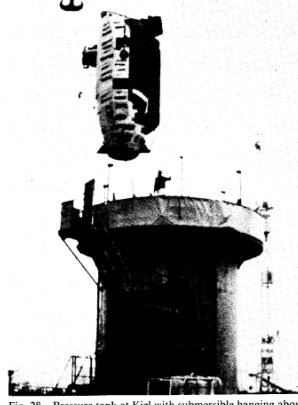
Fig. 28 – Pressure tank at Kiel with submersible hanging above
