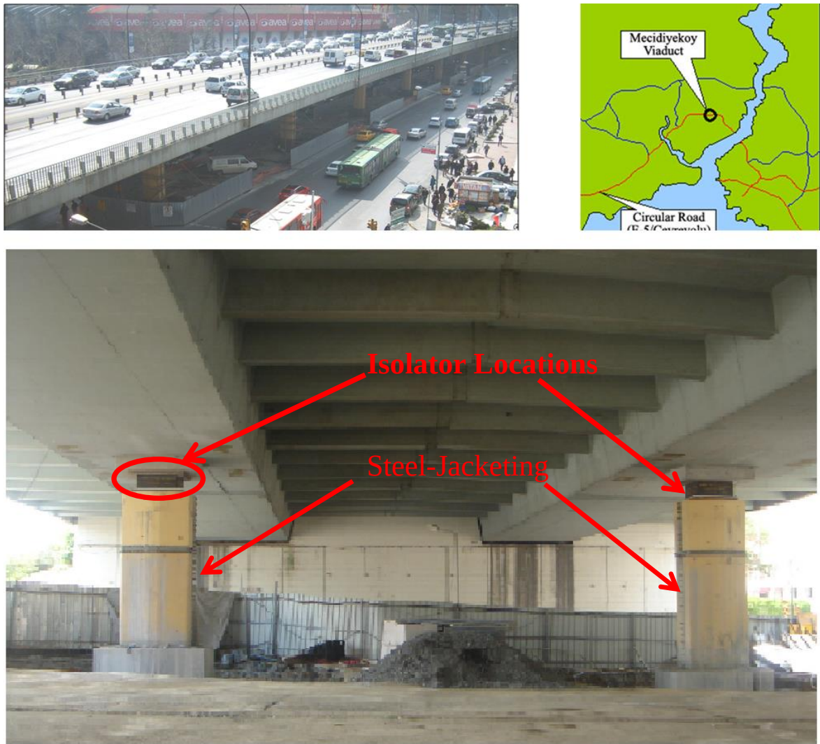
Figure 5.5. Location of Mecidiyeköy Viaduct and retrofit activities (Yenidogan and Erdik, 2014).
