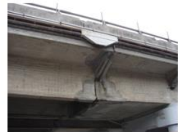
Figure 7.3. a) Cross section of the deck b) Gerber Saddles.
