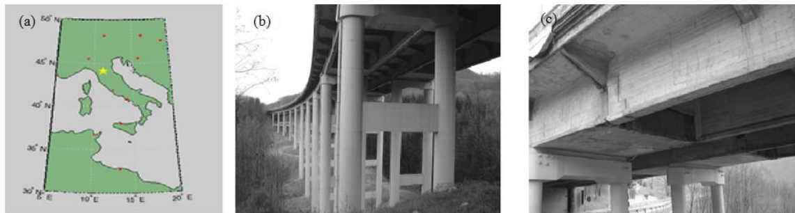
Figure 7.1. (a) Location of Rio-Torto Viaduct (b) General view of piers (c) Deck geometry.
