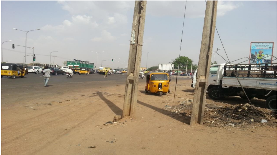
Figure 4.22 Improper poles location (Km 05+750) Bachirawa Junction-Airport Roundabout
