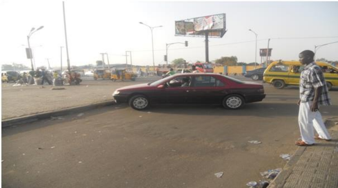
Figure 4.35 Inadequate turning radius at northbound approach
