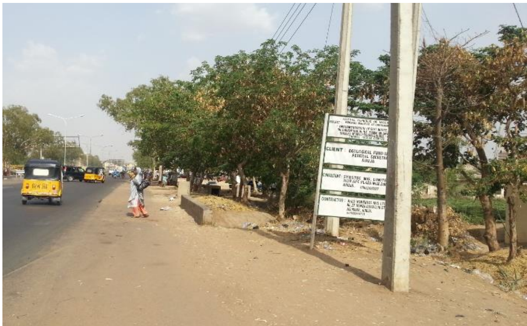
Figure 4.23 Improper pole locations (Km 07+200) Bachirawa Junction-Airport Roundabout Junction
