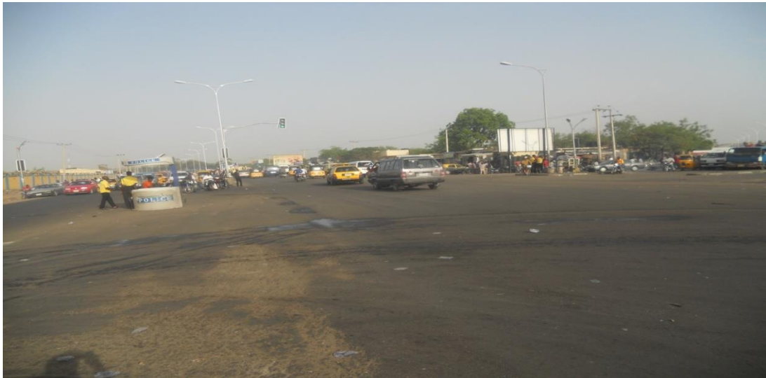
Figure 4.37 Lack of channelization
