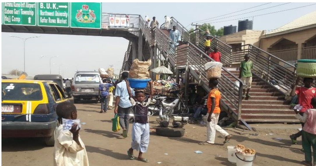
Figure 4.26 Improper pillar location (Km 04+900) Bachirawa Junction-Airport Roundabout
