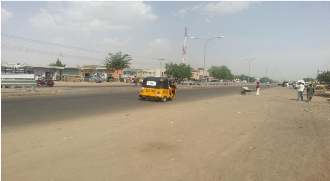
Figure 4.4 Absence of transverse marking (throughout the road section)
