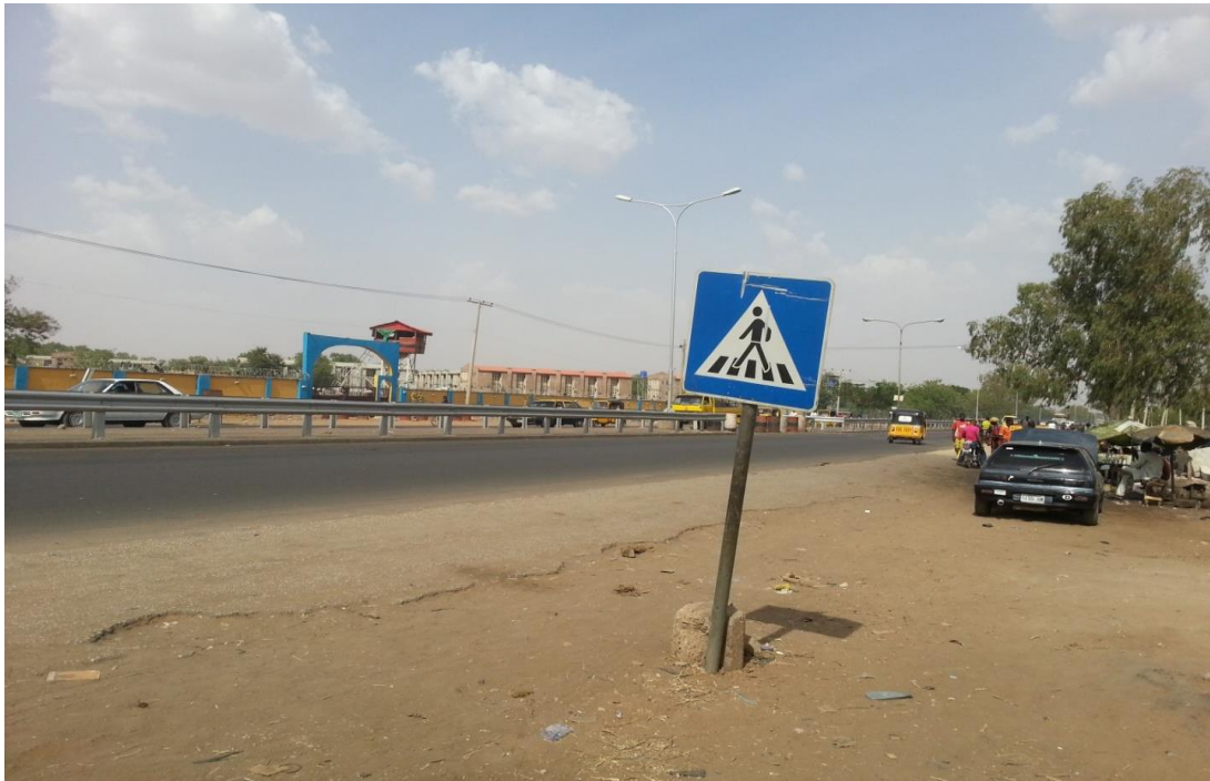
Figure 4.13 Improper pedestrian crossings (Km 06+550) Bachirawa Junction-Airport Roundabout
