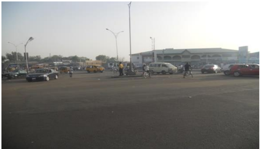
Figure 4.34 Lack of pavement markings at the intersection
