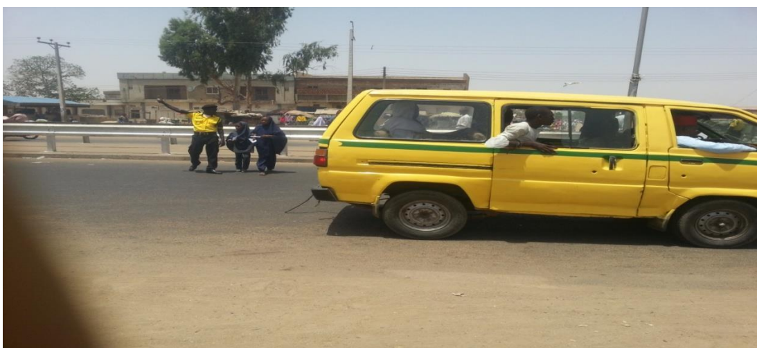
Figure 4.17 Lack of pedestrian crossing (almost throughout the road section)
