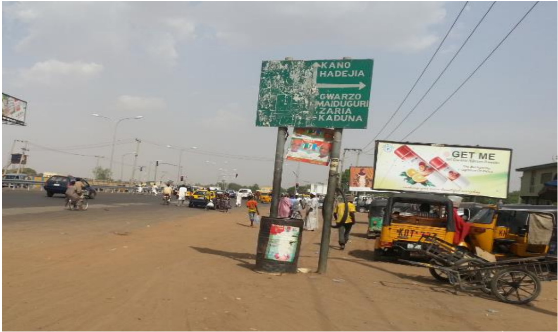
Figure 4.14 Worn out directional sign (Km 05+700) Bachirawa Junction-Airport Roundabout
