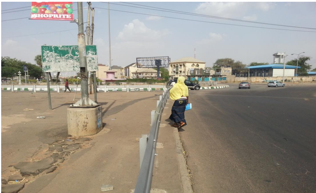
Figure 4.15 Worn out directional sign (Km 07+790) Bachirawa Junction-Airport Roundabout
