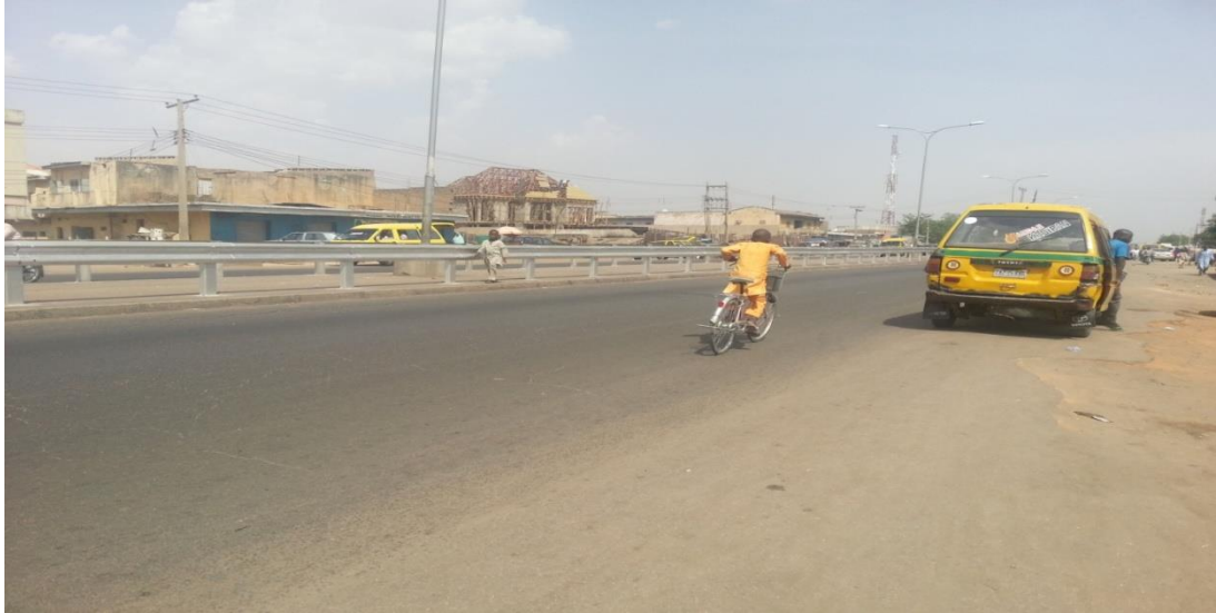
Figure 4.19 Lack of cyclist facilities (throughout the road section)
