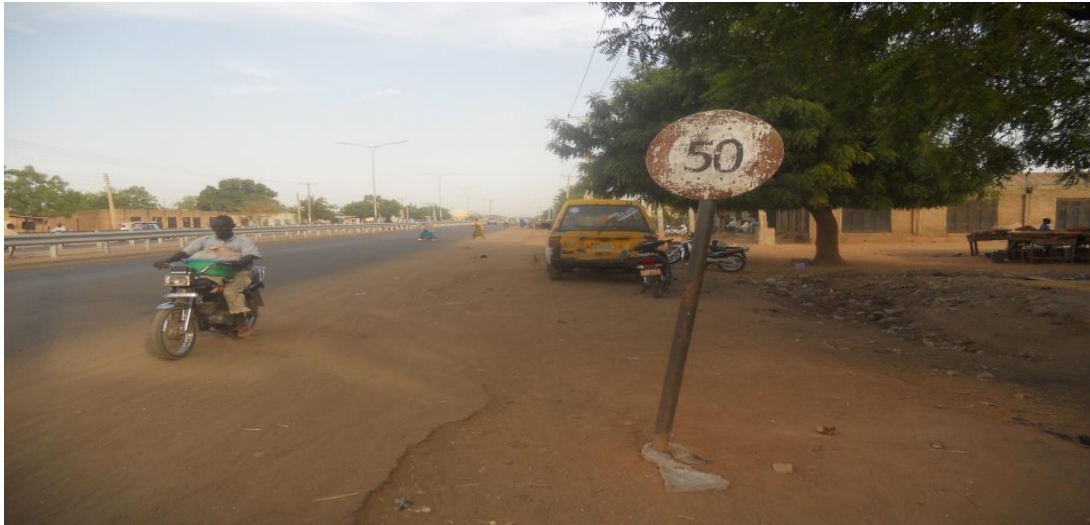
Figure 4.11 Worn out speed limit sign (Km 06+10) Bachirawa Junction-Airport Roundabout
