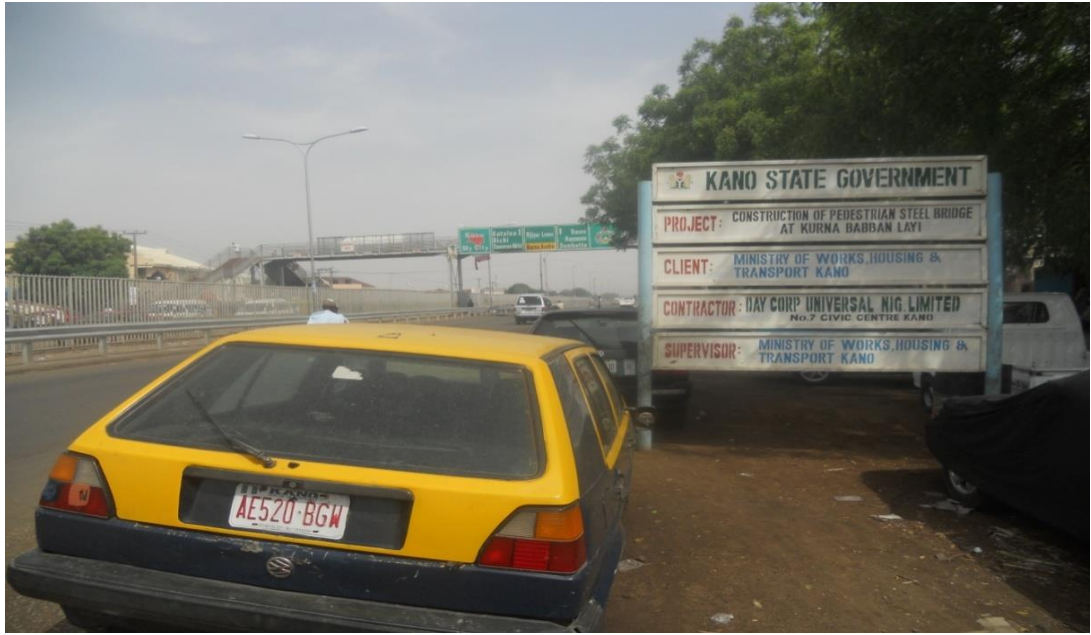
Figure 4.29 Improper signboard locations (Km 2+800) Airport Roundabout-Bachirawa Junction
