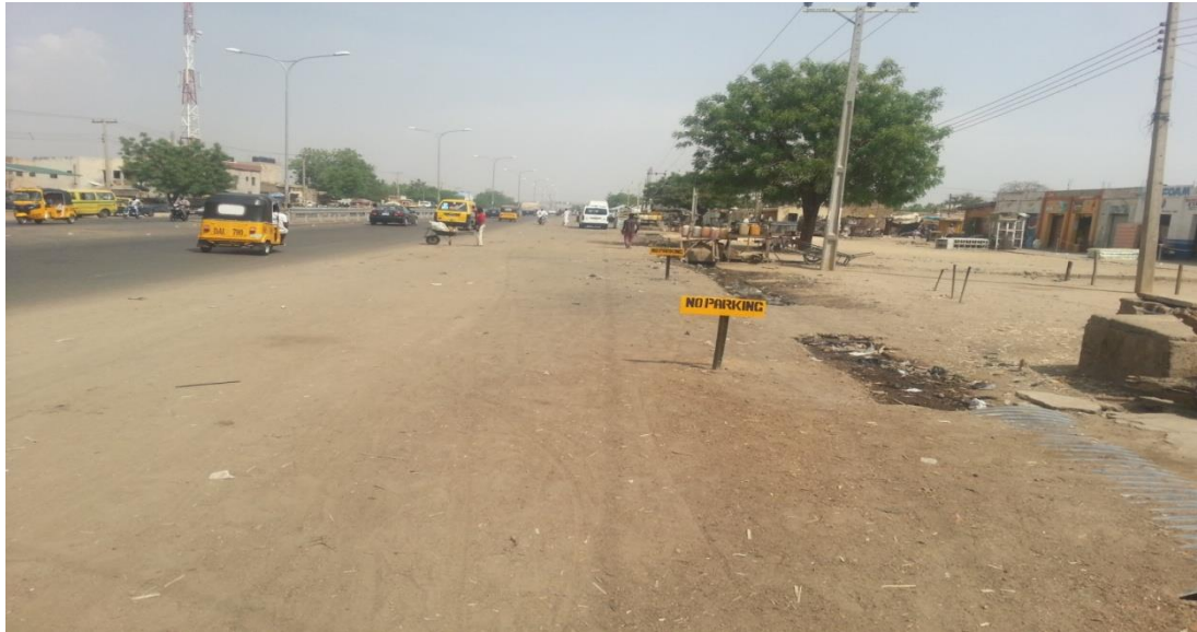
Figure 4.21 Improper parking controls (Km 03+500) Bachirawa Junction-Airport Roundabout
