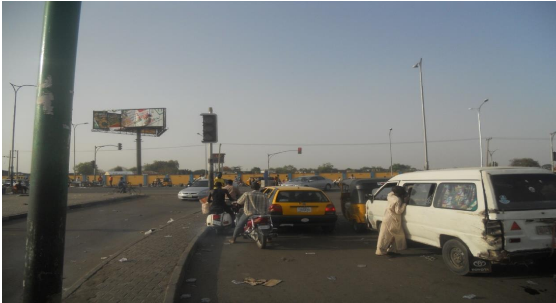
Figure 4.40 Lack of signal routine maintenance
