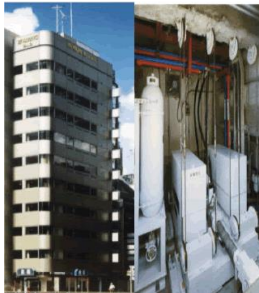
Figure 2.3 Kyobashi Seiwa building with active mass driver system (Gómez et al., 2007)
