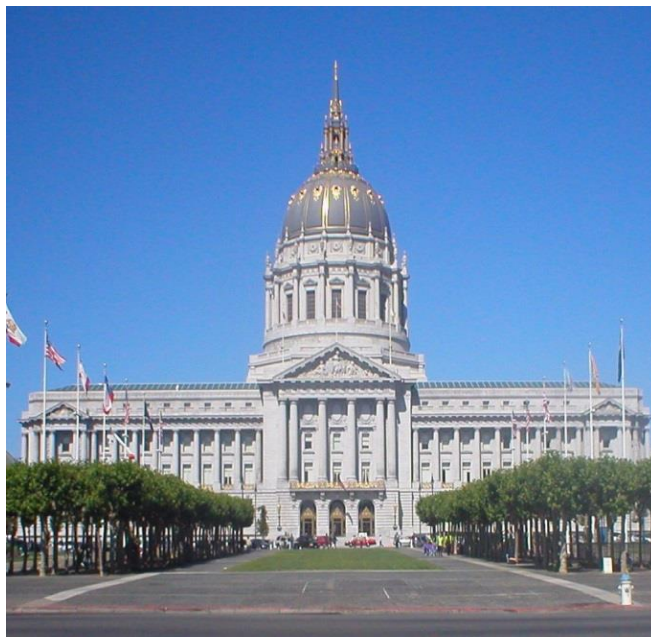
Figure 2.11 City Hall, San Francisco, California (Hofmann, 2011)
