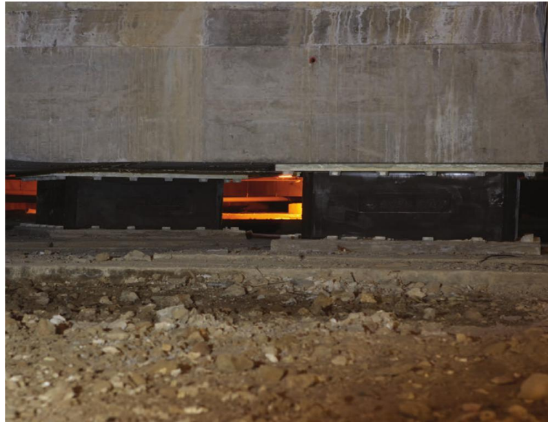
Figure 2.18 Lead rubber bearings used in the Museum of New Zealand (Stewart, 2012)
