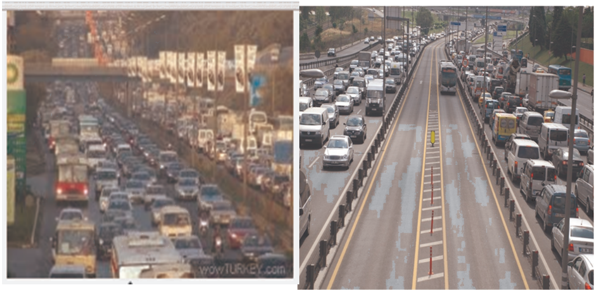
Figure 2.4. A view of D 100 Before Implementation of BRT Line on Left and After Implementation of BRT Line on Right in Istanbul (IETT).
