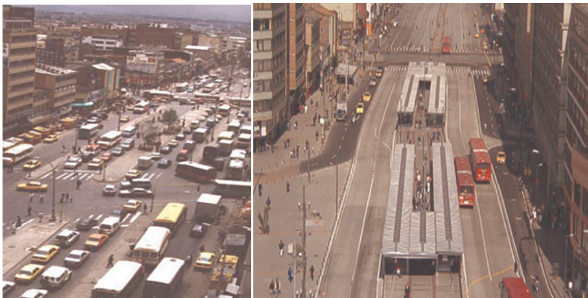
Figure 2.2. Bogota in 1998 Before Transmilenio on Left and Bogota in 2004 After Transmilenio on Right (Hamilton and Hidalgo 2004).
