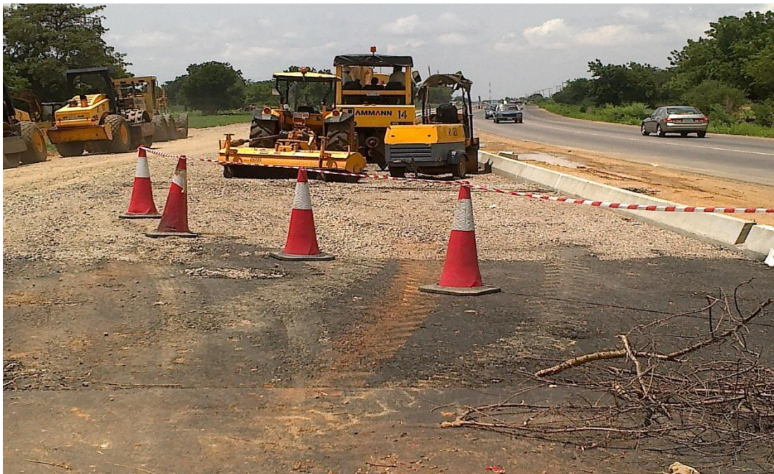
Figure D 4 Safe Keeping of Equipments After Work
