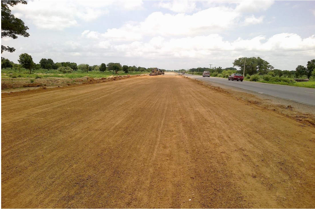
Figure D 3 Missing Buffer
