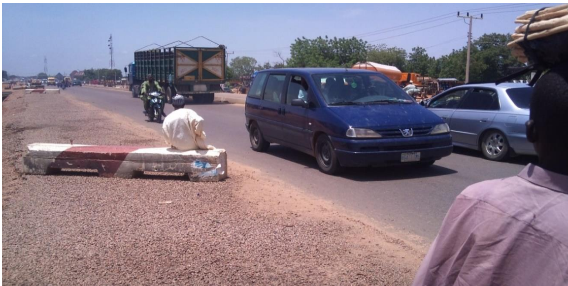
Figure 4-14 Misuse Of Traffic Control Device Km 3+450
