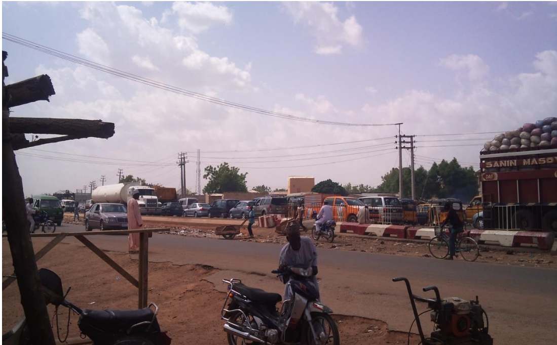
Figure D 1 Improper Access of users into Work Zone
