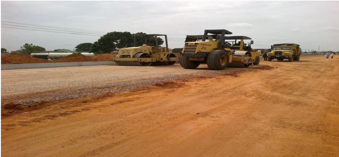
Figure 4-6 Missing Buffer Space Km 0+566
