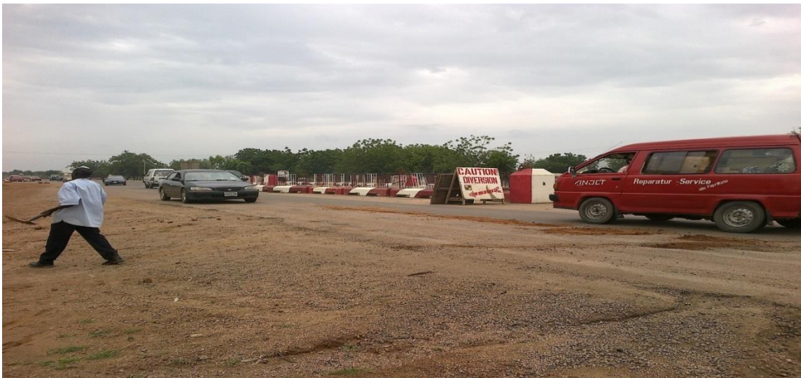
Figure 4-7 Missing Taper Km 9+500
