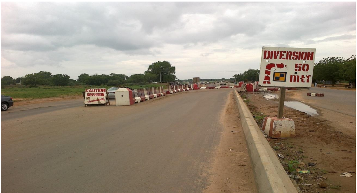
Figure 4-4 Confusing Traffic Signs Km 7+800
