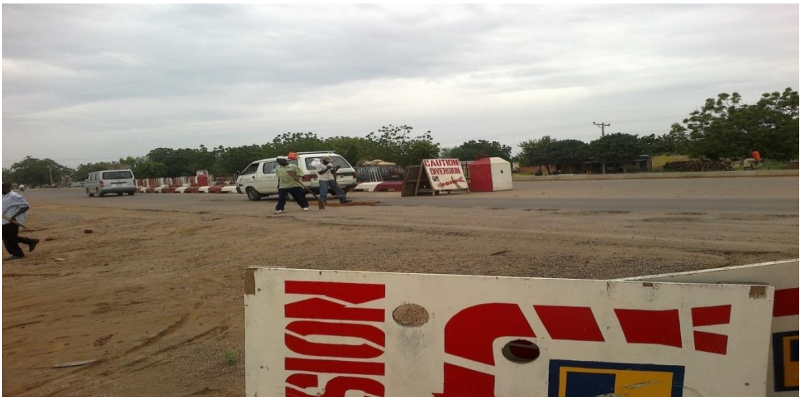
Figure 4-9 Worker Exposure to Moving Traffic Km 18+480
