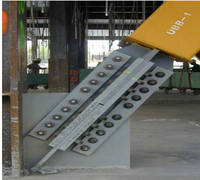
Figure 2.32 Standard bolted connection (Xie,2005)
