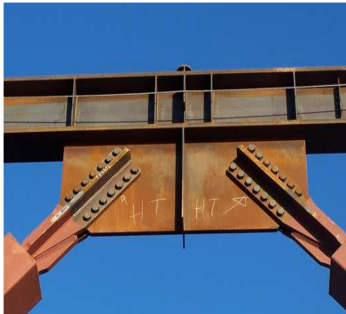
Figure 2.33 Modified bolted connection (Xie, 2005)
