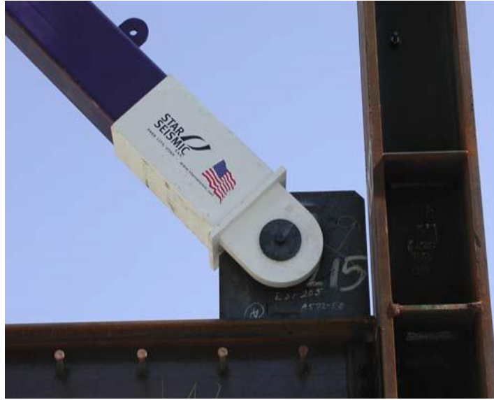
Figure 2.34 True pin connection (Xie, 2005)
