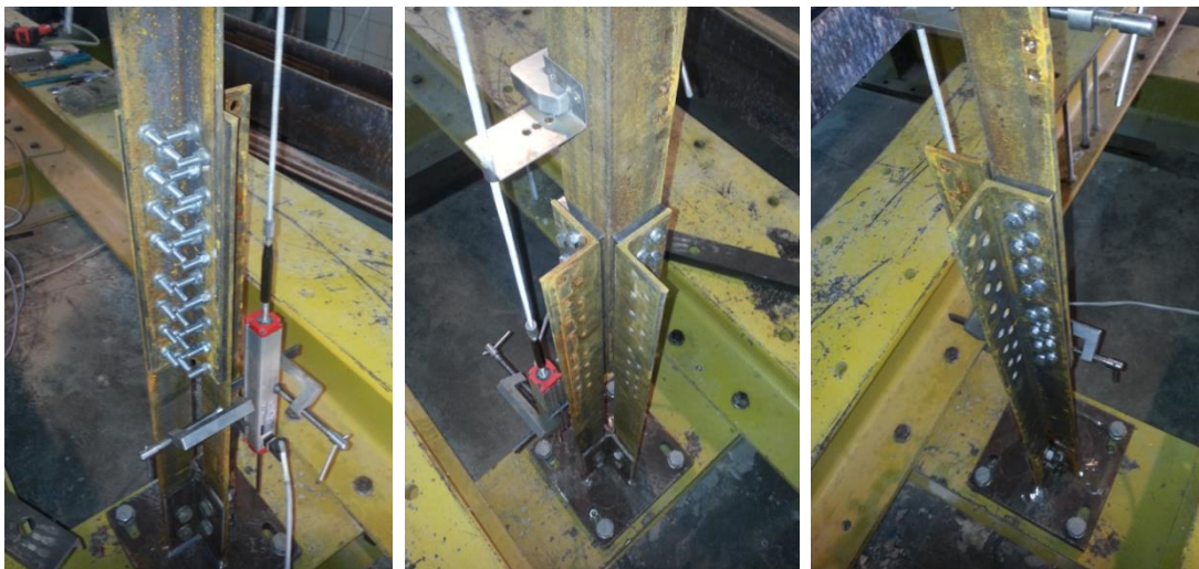
Figure 2.70. General view of Specimen-5
