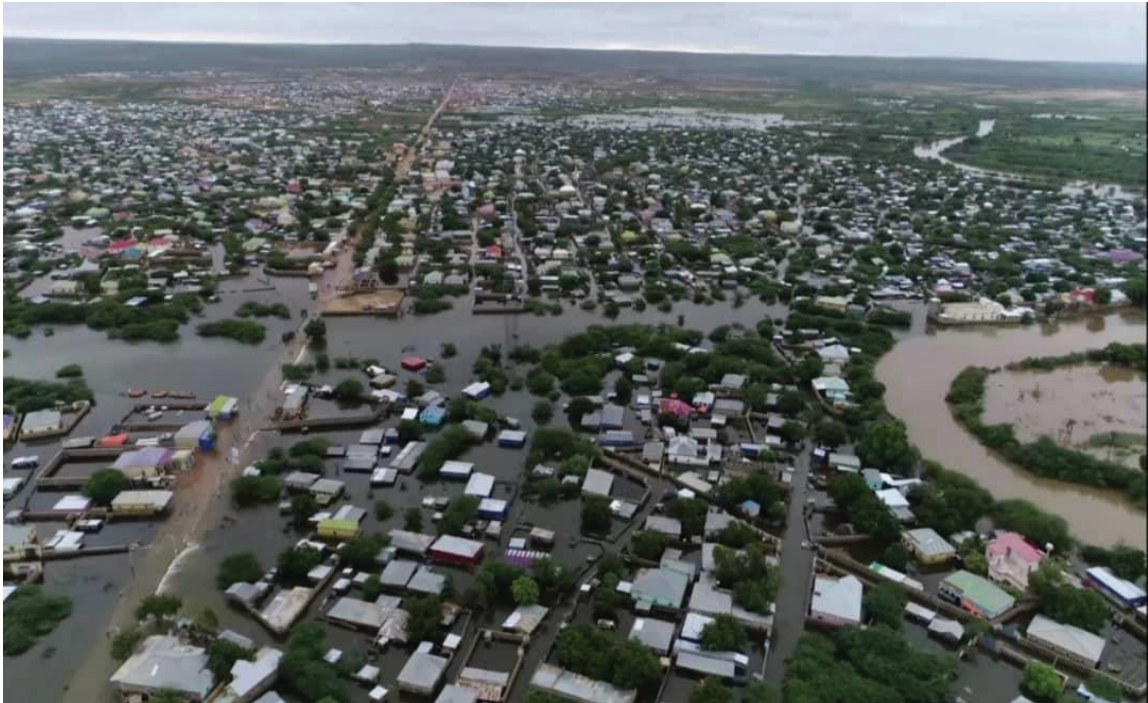
Figure 1.1. Flooding in Baledwayne City October 2019
