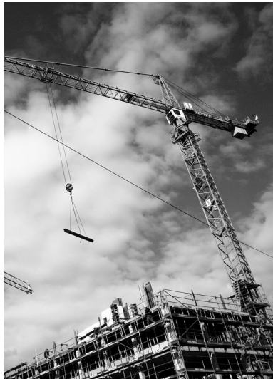
Figure 2.1. Construction crane operations, Rübiger (2011).
