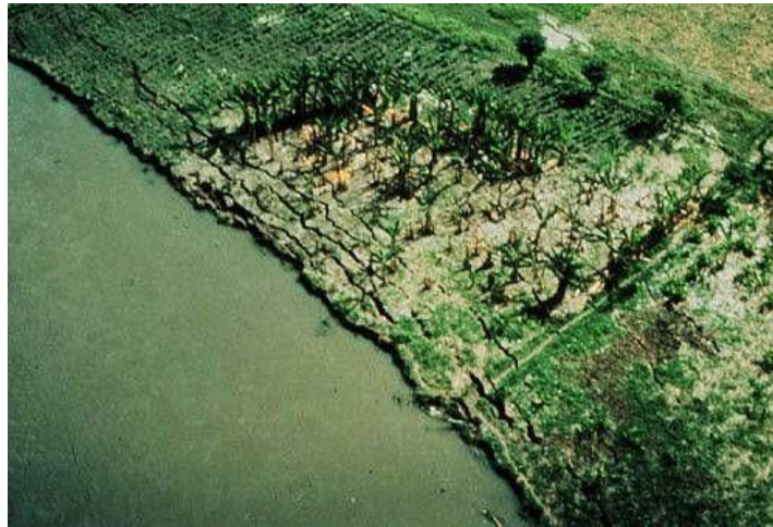
Figure 2.4. Motagua Riverside ground cracks in 1976 Guatemala Earthquake
