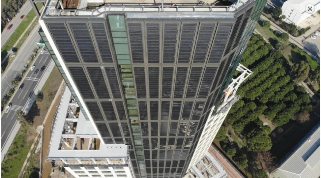
Figure A1.7. İstinye Park SPP- İzmir BIPV (Building - Integrated PV) (From gtctrade.com)
