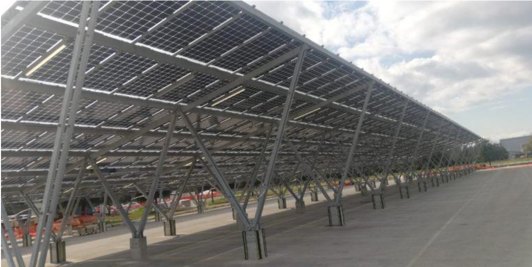
Figure A1.11. TAV Muğla Airport SPP. Project Type: Bifacial Carpark (From gtctrade.com)
