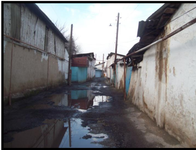
Figure 4.13 A View from A Type Tashkent Mahallas
