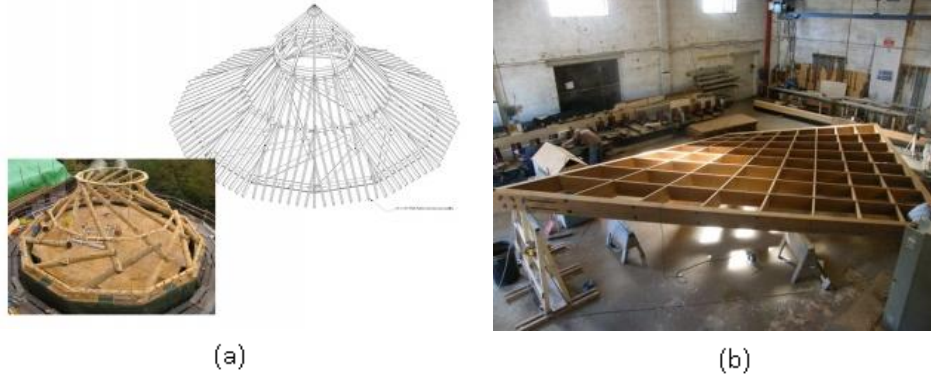
Şekil 5.26 Hiperbolik paraboloid sistem kurulumu (a) Hill Holt Woodland Centre ve (b) Gillespie Hyperbole [137]
