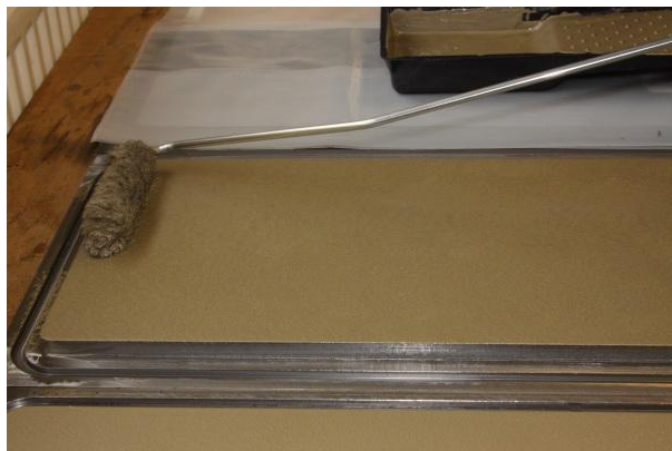
Figure 6.4 : The application of anticorrosive with roller.
