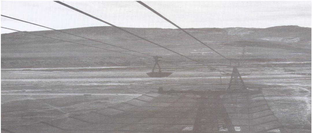
Figure 75: Transportation of the Broken Ores from C Placer to Demirdağ Station by Aerial Ropeway (1942-1985)
