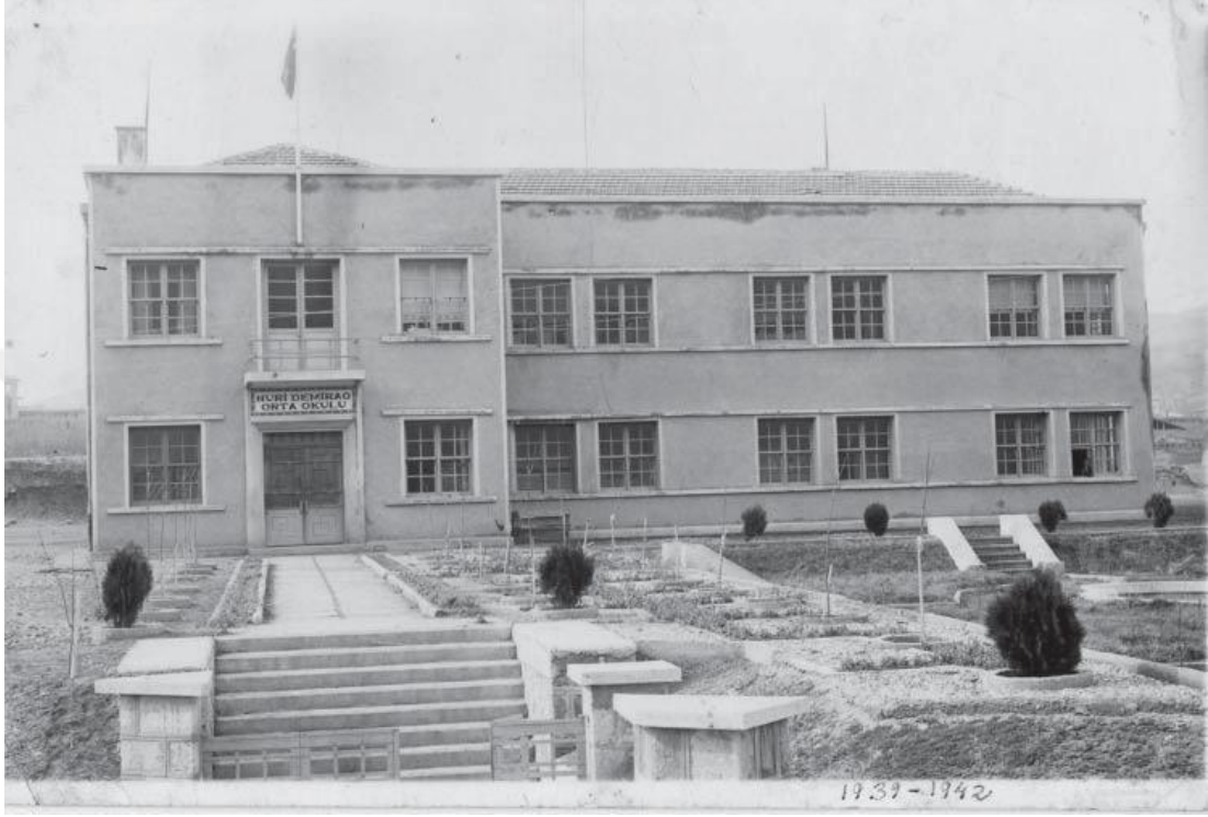
Figure 13: Nuri Demirağ Secondary School
