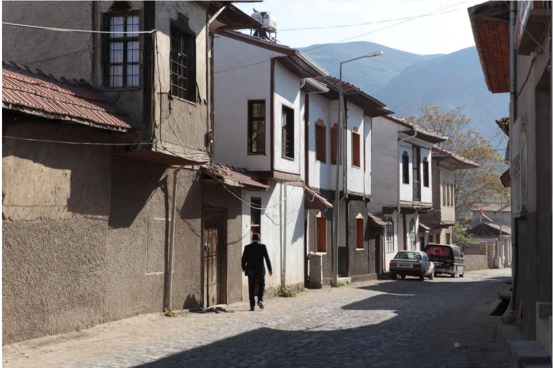
Figure 34: Traditional Two-Storey Houses
