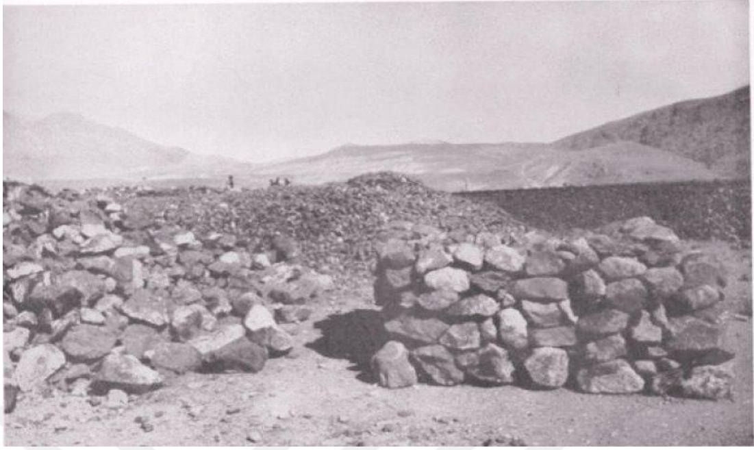
Figure 69: Iron Ores Stored at Divriği Station in the 1940s
