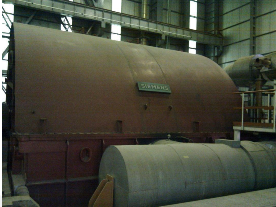
Figure 2. 11 Steam turbine of NG-CCPP [24]
