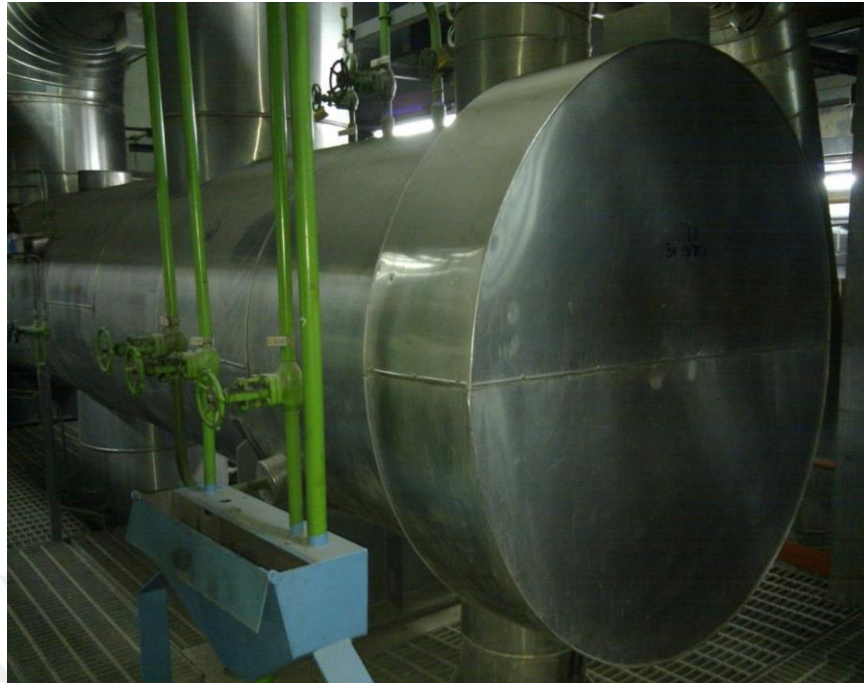
Figure 2. 9 Feedwater tank of NG-CCPP [24]
