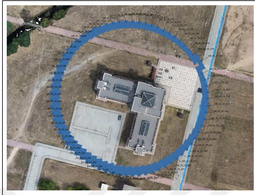
Figure 4.6: A set of aerial photos captured in circular flight mode for aerial photo orientation using the SfM method.
