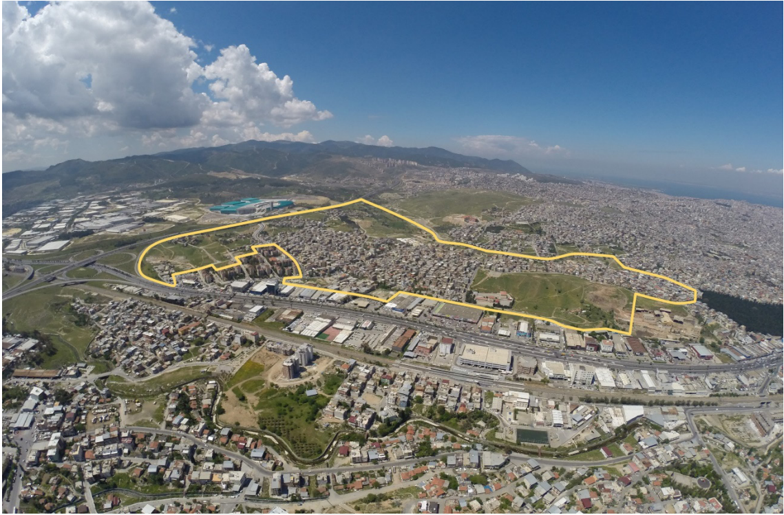
Figure 4.4. Photograph of the case from east direction
