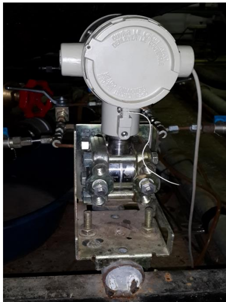
Figure 20. Honeywell ST 300 Differential Pressure System
