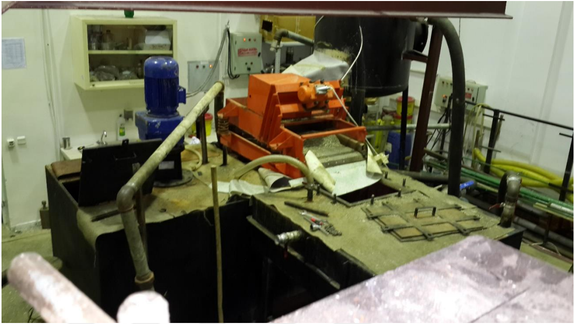
Figure 30. A View of Liquid Tank, Solid Separation System and Collection Tank
