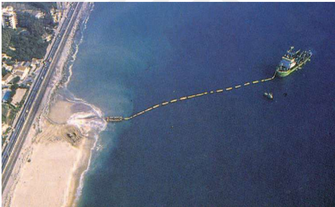
Figure 4.1 : The dumping of dredged material through pipeline for beach nourishment (Vidal et al, 2010).
