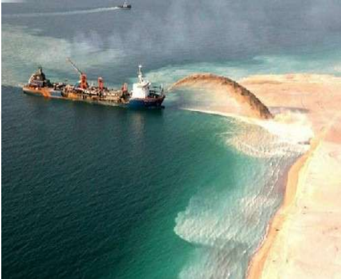
Figure 3.3 : The dumping process of land reclamation ( http://onyxresources.onyxgoc.com/ ).
