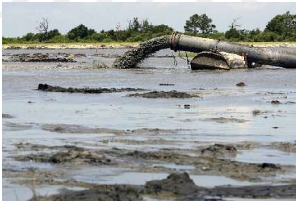
Figure 4.2 : The dumping of dredged material through pipeline for marsh nourishment ( http://www.nola.com ).
