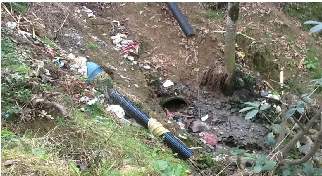
Figure 2.6 : Sewer Pipes and Discharge Point to River at Dikkaya Village.
