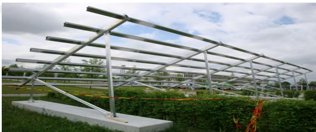
Figure 3.2 : Aluminum construction of a PV system.
