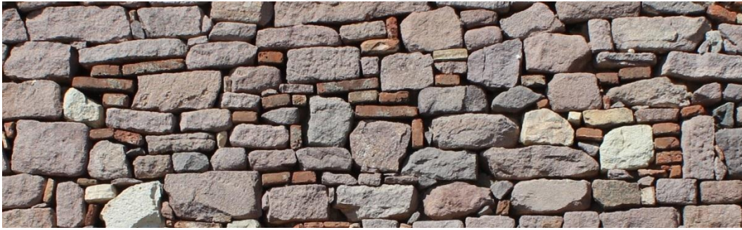
Figure 54 A typical rough cut masonry pattern in Ildır (taken by the author)
