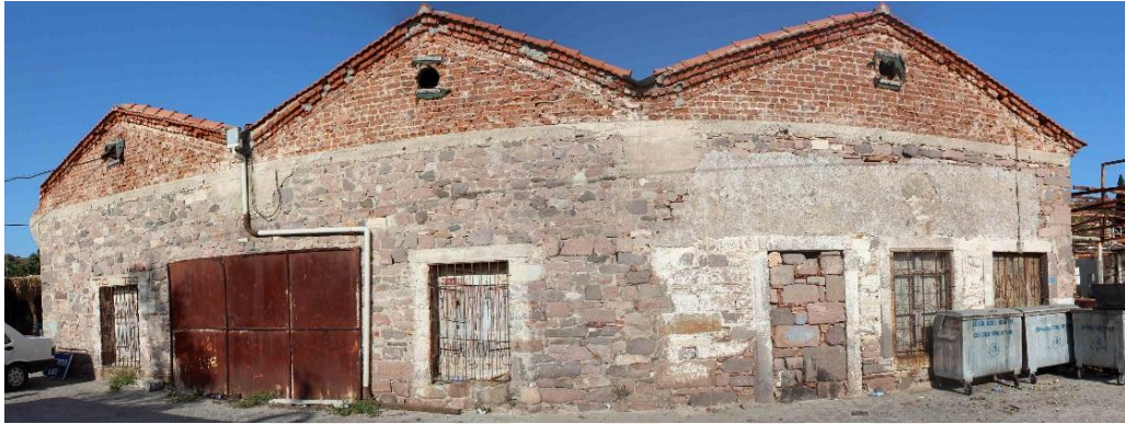
Figure 70 Olive Oil Factory (taken by the author)
