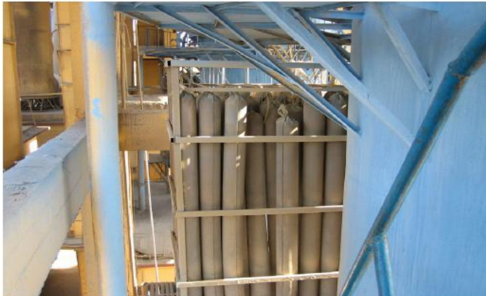
Figure 4.5. Bag filters used to clean gasses in VSKs (Viacrozc,2005).
