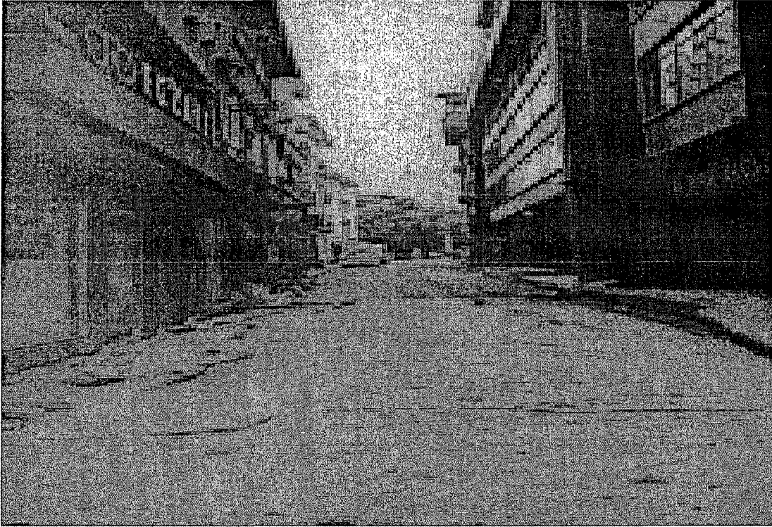
Figure 2-7 Liquefaction-Induced Settlement of Adjacent Buildings and the Uplift of the Sewage System Pipe (NZSEE, 1999)
