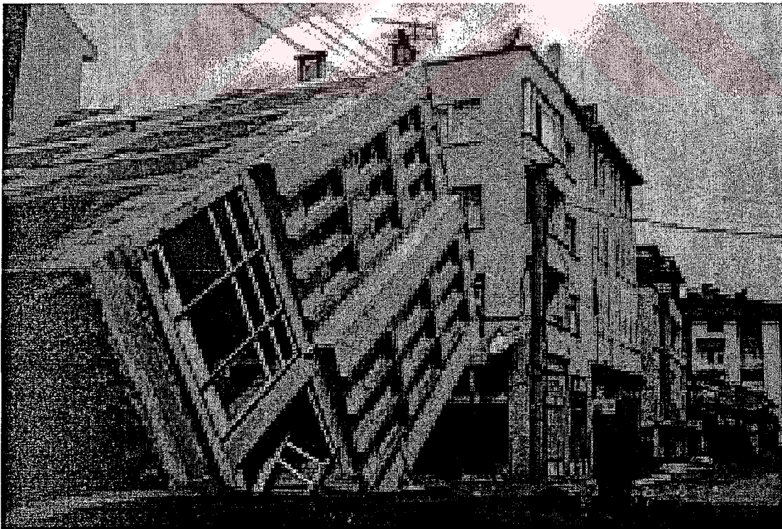
Figure 2-8 Tilted and Collapsed Buildings in Adapazarı (NZSEE, 1999)
