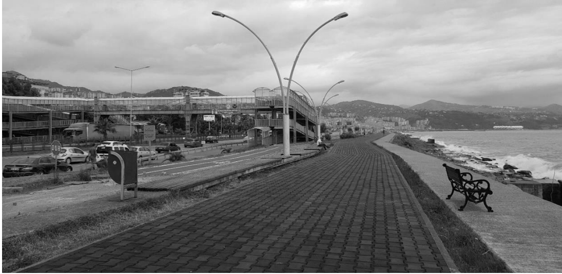
Figure 62: An overpass on the coastal highway (Source: the author, 2019, July 14)
