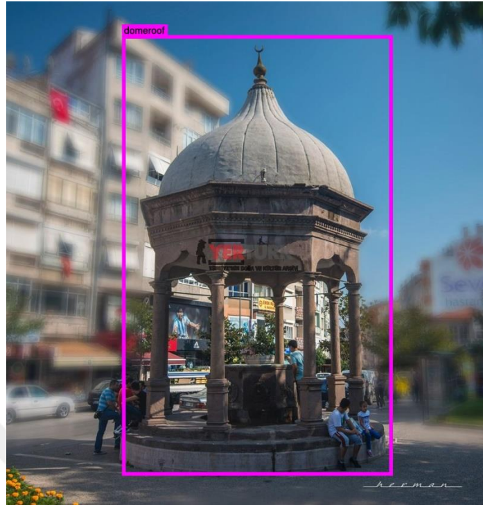
Figure 5.3 Detection of Fountain with Dome Roof 1
