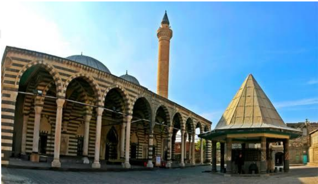
Figure 2.3 Diyarbakır Behram Paşa Mosque Fountain [17]
