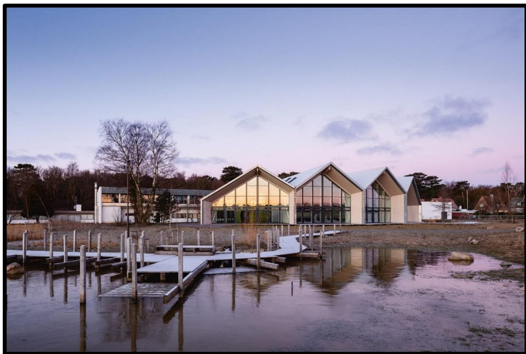
Figure 3.18: Shows the Facade of Conference Hall and Hotel by Green Solution House in Denmark (GXN, 2015).
