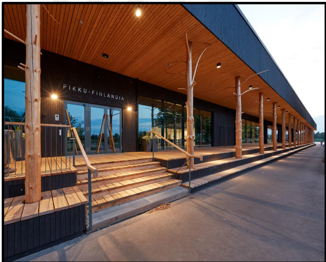
Figure 3.3: Shows a Photo by Kimmo Raisanen to the Little Finlandia in Helsinki Is a Modular Conference Venue Held Up by Pine Trees as an Example of Circular Design which Aims to Use and Reuse Materials without Harming the Environment by Manufacturing and Creating Too Much Carbon Emissions (Barker, 2022).
