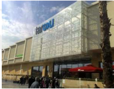
Fig. 6-20: (Left) Main entrance from the Adana Boulevard
