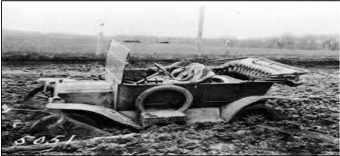
Figure 1.1: Old Roads Problems[2] .
