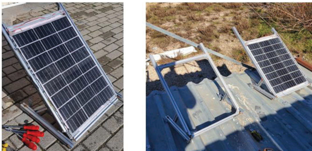
Figure 2.25 The laminated PV module and produced mechanical frame for the adjustment of the tilting angle.
