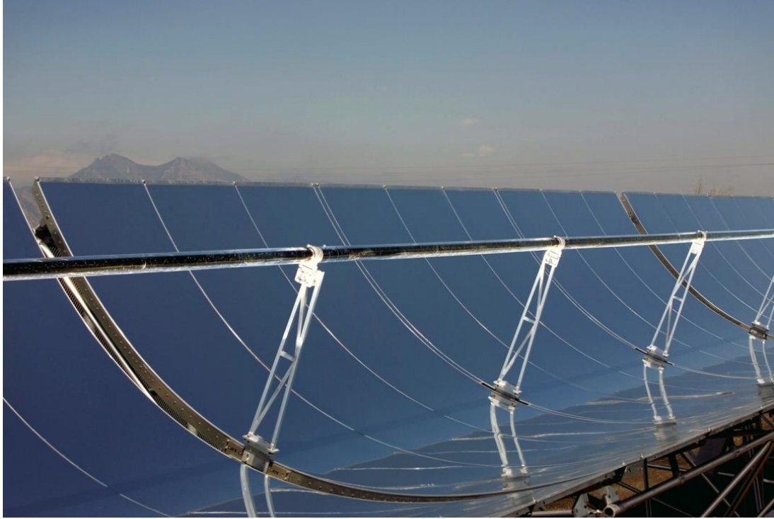
Figure 2.4: Parabolic Trough Collectors [19].
