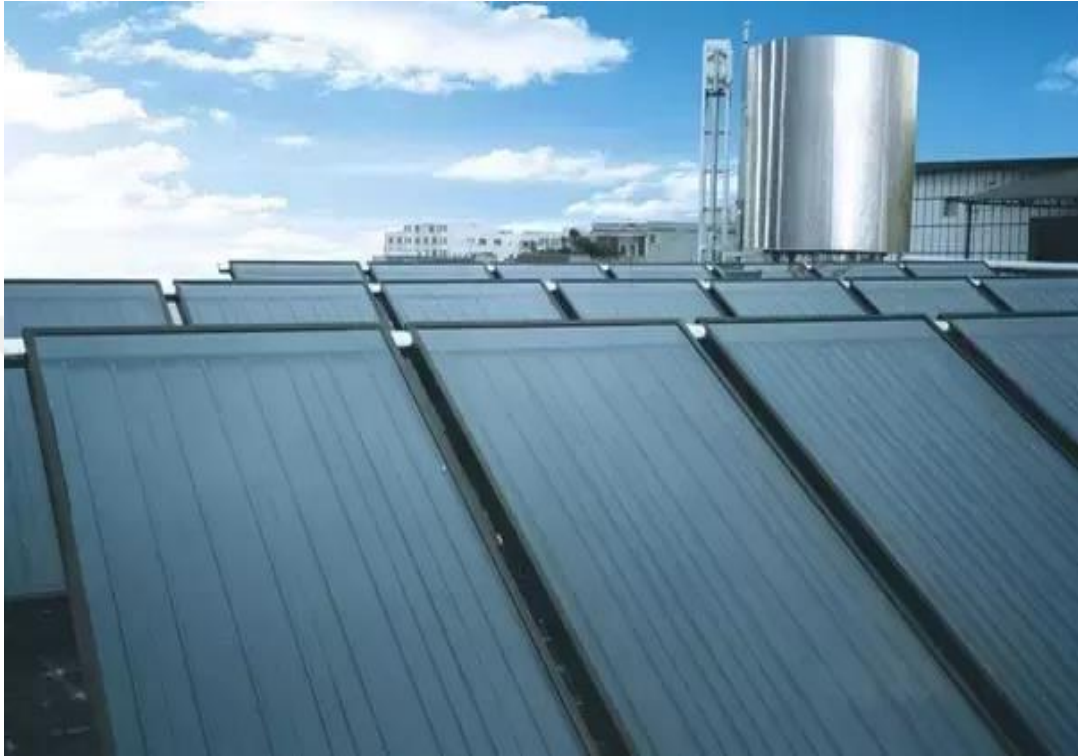
Figure 2.2: Flat Plate Collectors [14].
