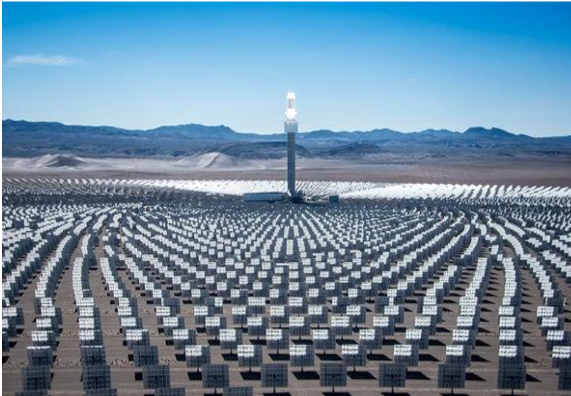
Figure 2.7: Heliostat Field Collectors [23].
