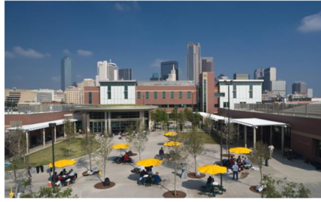
Şekil 2.28. “The Bridge Homeless Assistance Center”, avlu (Rosenberg 2011)
