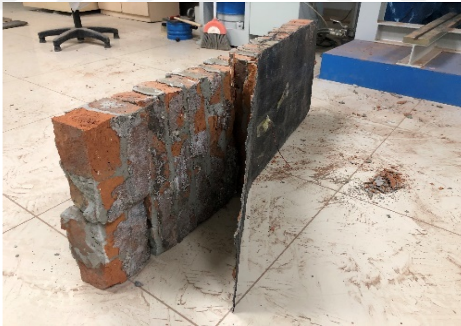
Figure 4.16 Testing & Failure mode of S-F-L1
