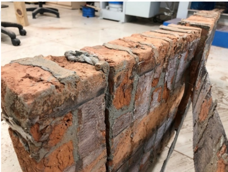
Figure 4.14 Testing & Failure mode of S-S2-L3
