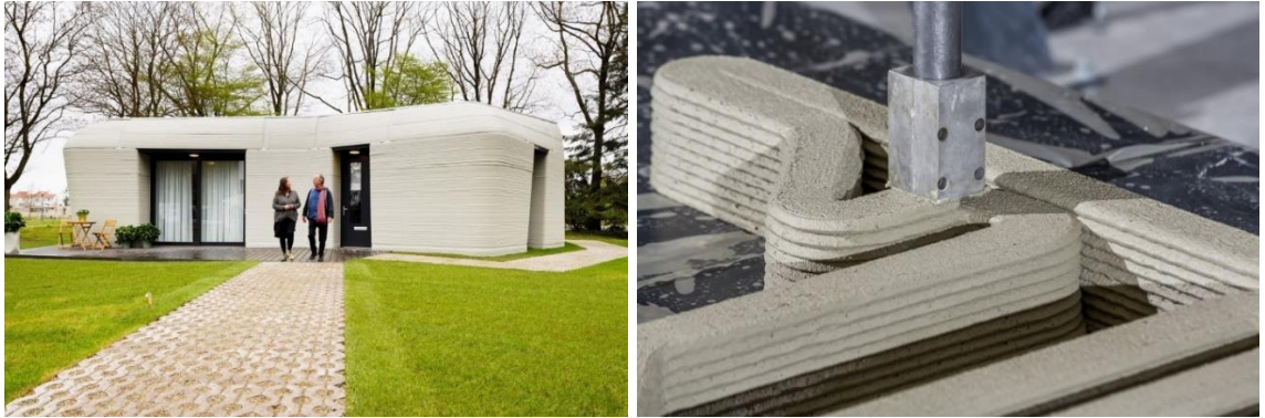
Şekil 4.17. Project Milestone, 3D beton baskıya dayalı ilk ticari konut projesi, Eindhoven University of Technology ve Studio Houben & Van Mierlo Architecten (URL-4.10)
