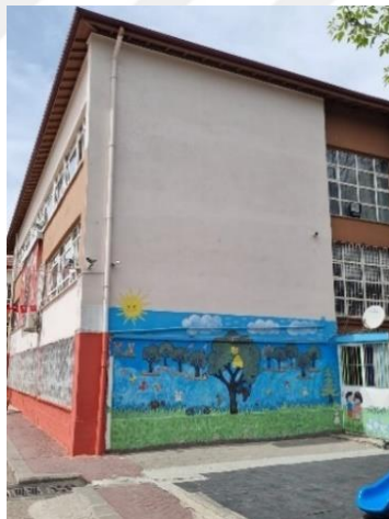
Figure 2.19. Painted walls of the children’s garden at a school.
